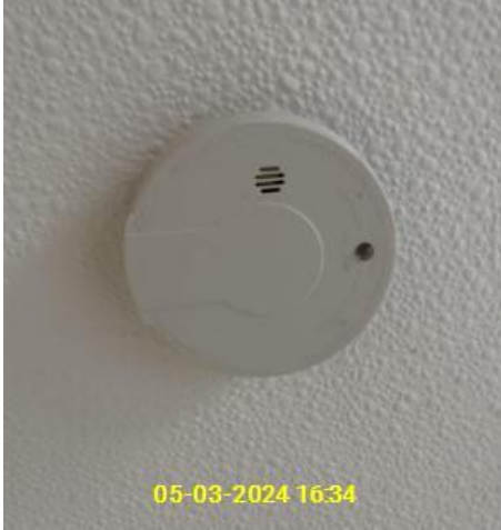
4.1.1 - Smoke Alarms - condition
