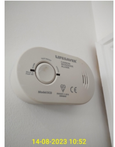
5.2.1 - Alarms - carbon monoxide detector
