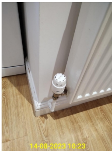
8.14.1 - Kitchen - heating Thermostatic radiator valve (TRV).
