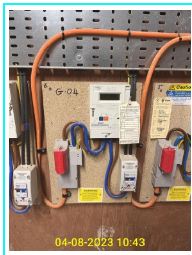
2.1.2 - Meters - electricity meter
