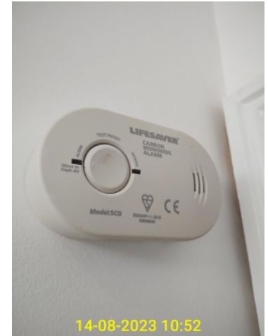
5.2.1 - Alarms - carbon monoxide detector
