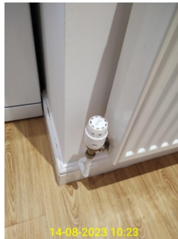
8.14.1 - Kitchen - heating Thermostatic radiator valve (TRV).
